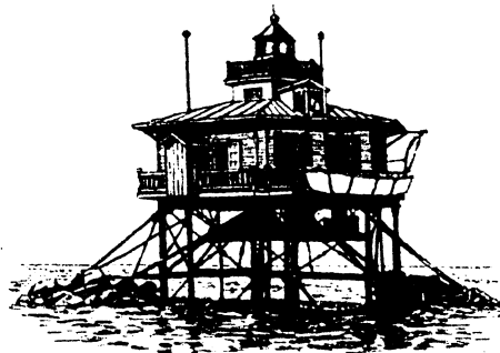
Figure 8 Windmill Point Lighthouse at the Mouth of the Rappahannock Supported on Wrought Iron Screw Piles (similar to lighthouses in the Delaware Bay) (Snyder & Guss, 1974).
